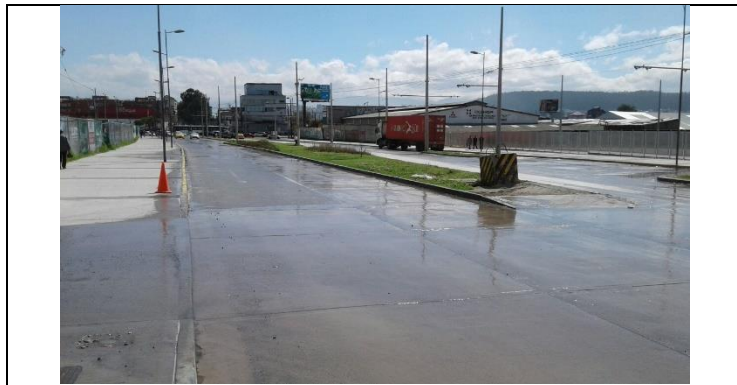
Central Dovelas Norte-TBM
