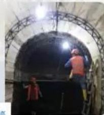
TUNEL GALO PLAZA
