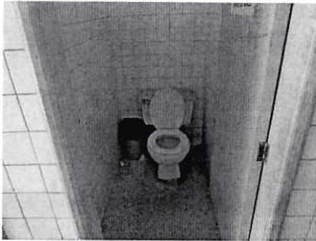
Baños vista interior
