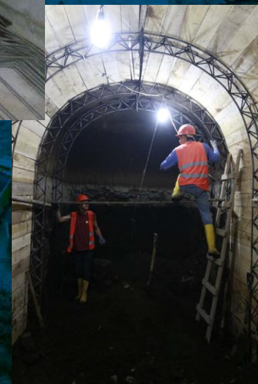
FIG.19. TUNEL GALO PLAZA - 2018
