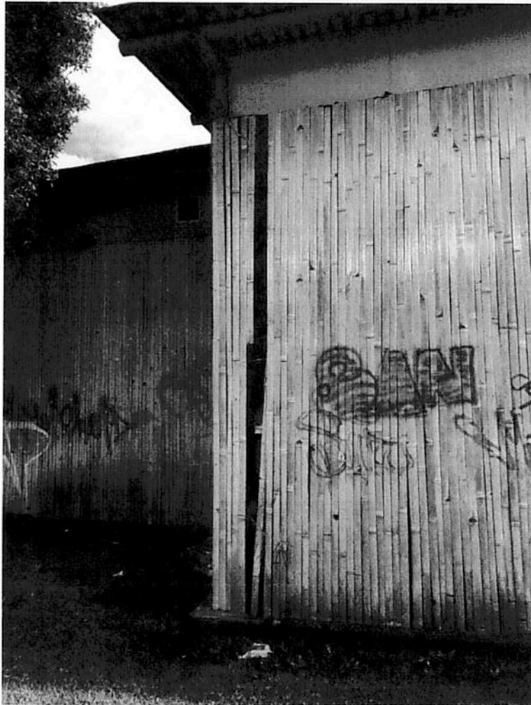
FOTOGRAFÍA 12: RECUBRIMIENTO DE CAÑA EN PARED EXTERNA
