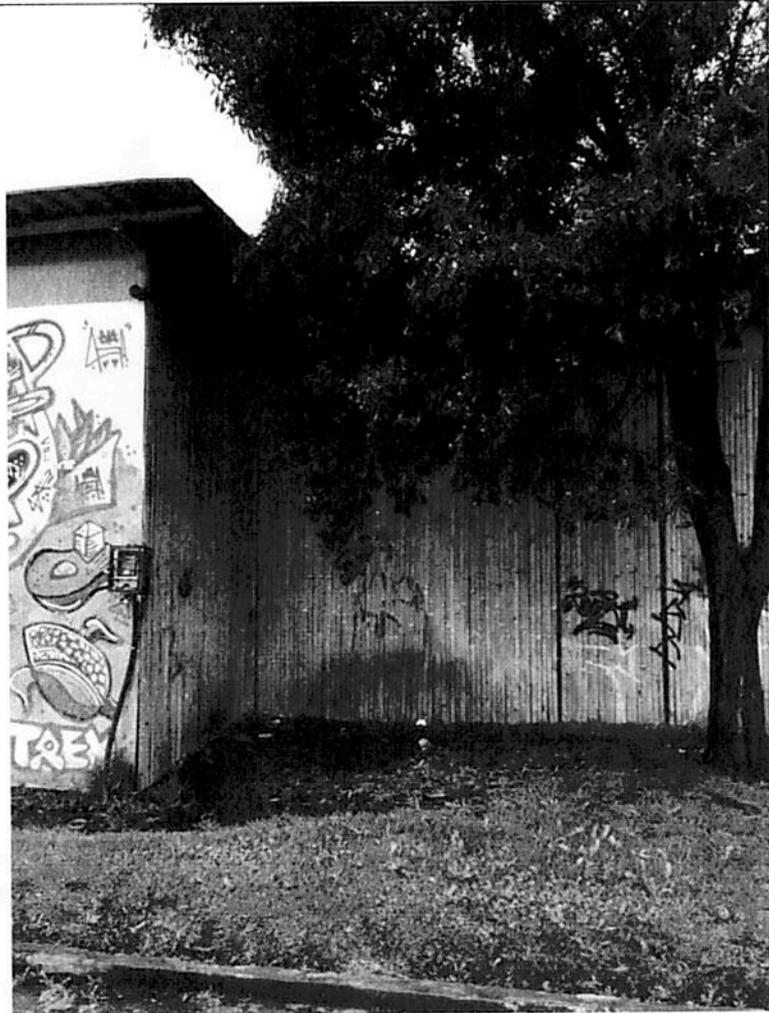
FOTOGRAFÍA 13: RECUBRIMIENTO DE CAÑA EN PARED EXTERNA
