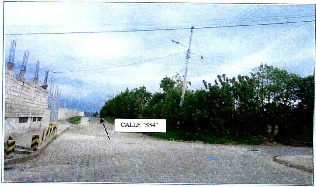
CALLE "S54" : (TRAMO FINAL)
